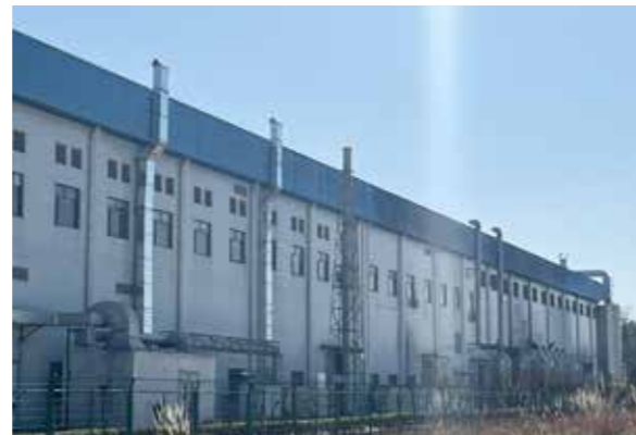
Exhaust treatment facilities of Li-ion battery factories
