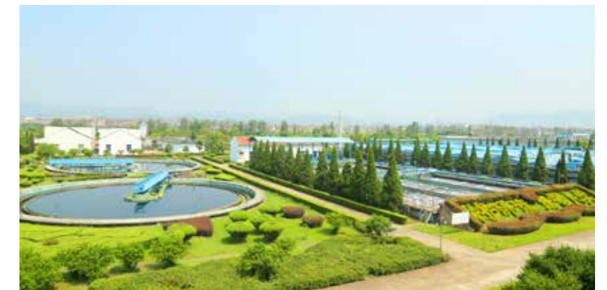
Wastewater treatment stations
